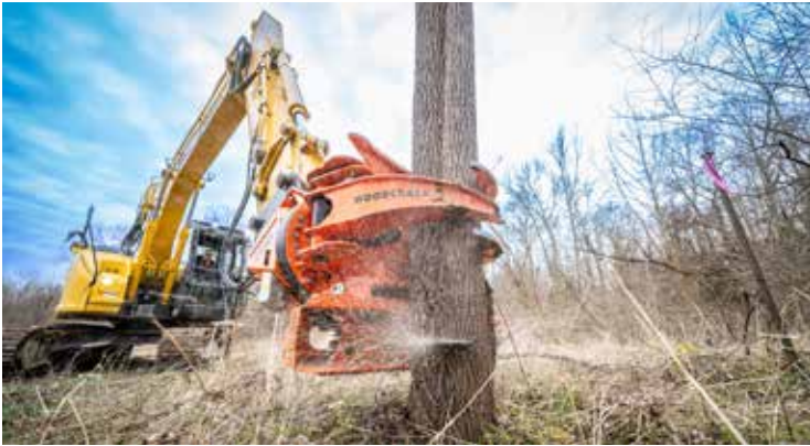
Maintenance work along traffic roads.
