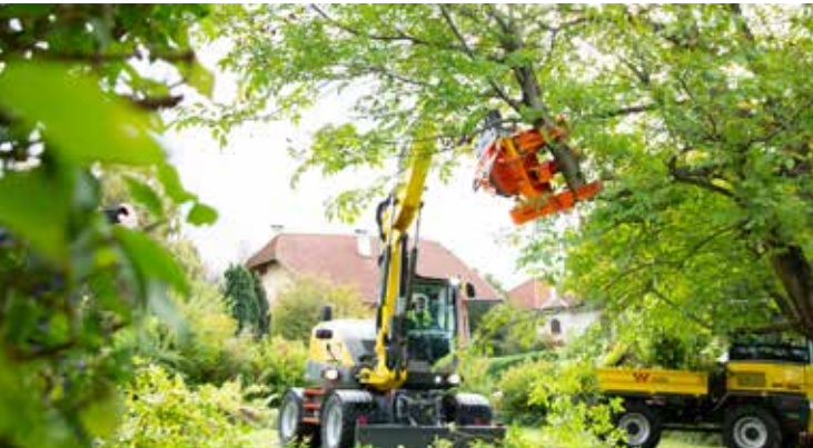
C250 at the wheel excavator.
