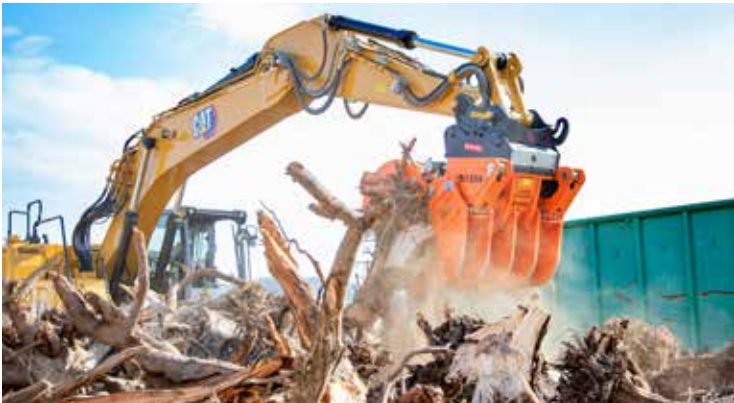
Clearing and caring of large areas.
