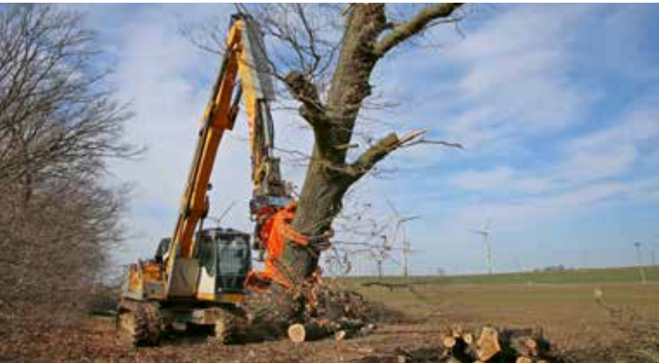
Maintenance work along traffic roads and routes.
